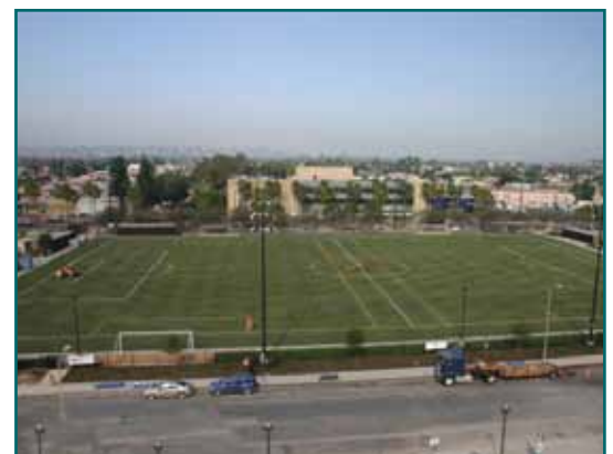
Expo Center Sports field after renovations
