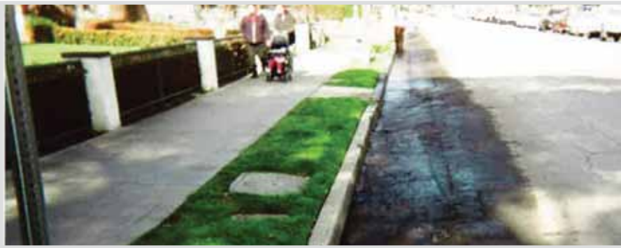
28th Street after clean-up
