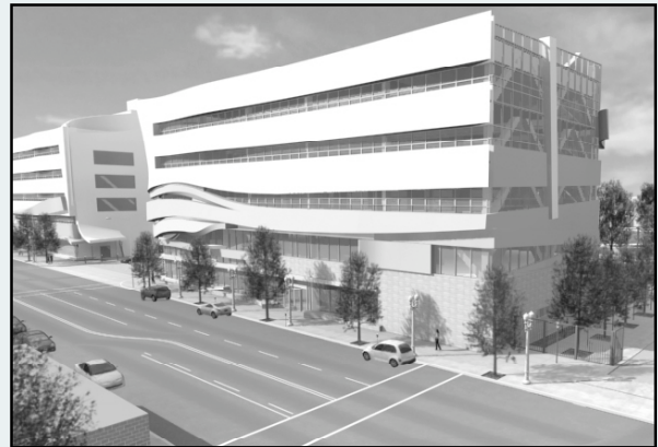
Construction on the LATTC's $77 million South Towers at Grand Ave. and 23rd St. will begin this fall. The buildings will include some "green" elements.
